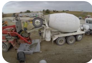
Concrete Batching Services
