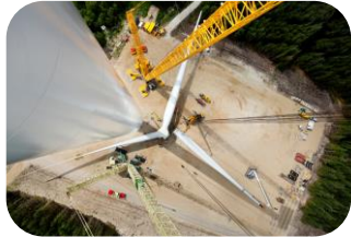
WTG Installation Up to 226
