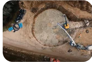
WTG Foundations Up to 226
