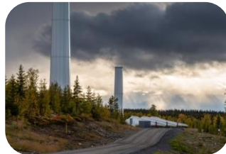
Road Upgrades Up to 250km
