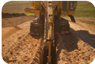
Underground Power Cable Install
